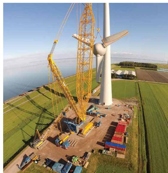
Park in the Netherlands, using a 1,650 tonne capacity Terex CC 8800-1 lattice boom crawler crane, equipped with the new Boom Booster, a boom structure increasing the lifting capacity.
