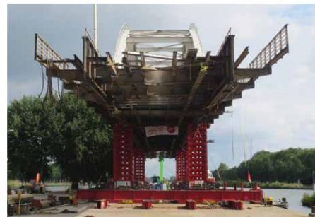
Mega Jack system, that has a capacity of 5,200 tonnes per tower.
